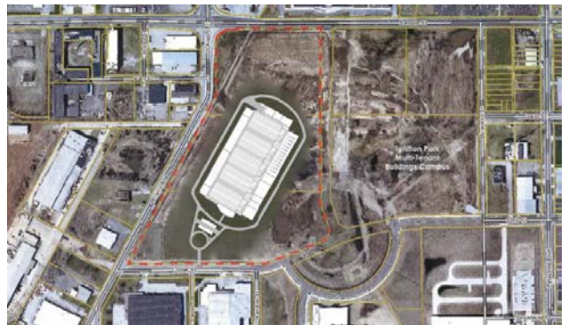
View of 100,000 square foot data center on site
