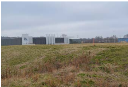
View from east corner looking southwest
