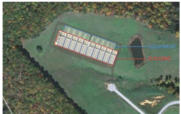
Aerial view of data center at site
